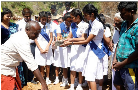
Building public latrine facility for the Namunukula Estate Community
